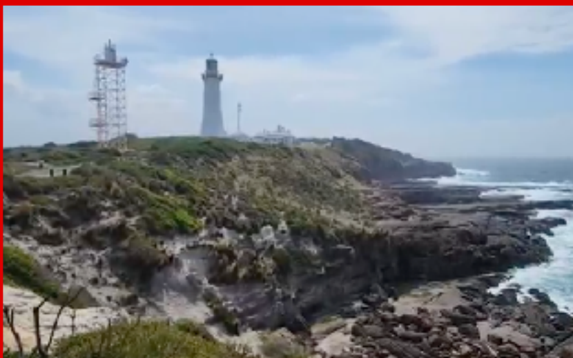
Green Cape Lighthouse and the new light tower.
